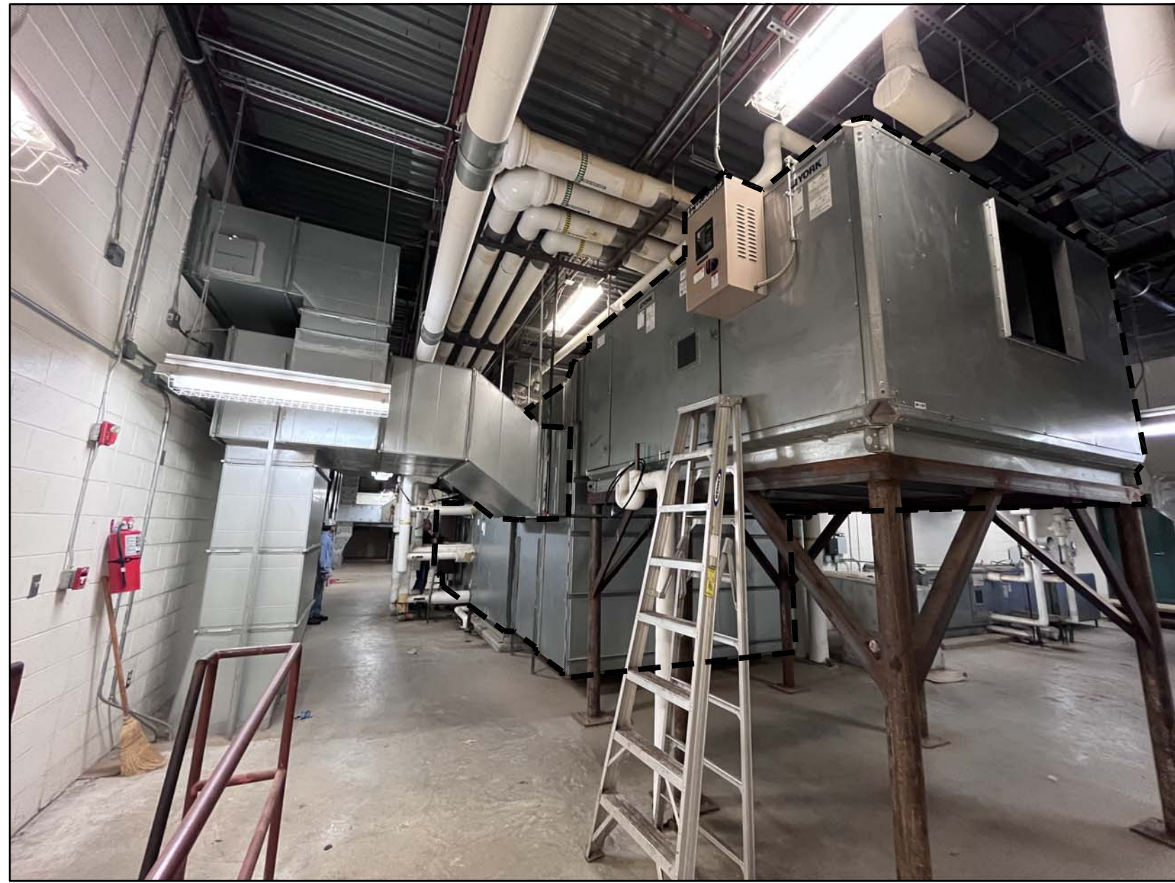
P12 AHU-2 AND AHU-2A EXISTING CONDITIONS
