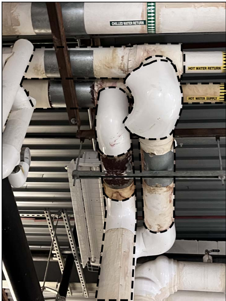
P16 DAMAGED HOT WATER PIPE INSULATION (TYP)
